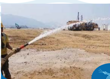
工人定時向工地灑水 Workers regularly hose works area
