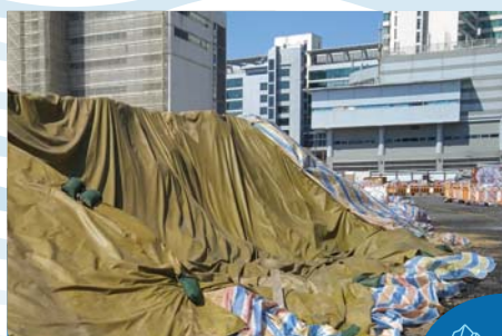
以不滲透的隔塵布覆蓋儲料區 Covering stockpiling areas with impervious sheets
