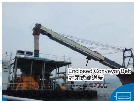
使用封閉式輸送帶運送填料 Using enclosed conveyor belt to transport fill materials
