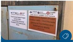
利用不同顏色的標籤 · 協助工友分辨在限制和非限制時段內使用的機動設備 Coloured labels on Powered Mechanical Equipment (PME) for site workers' easy differentiation between equipment for use in non-restricted hours and restricted hours
