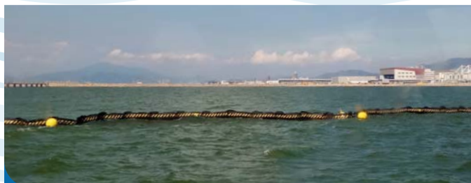
除局部設置的淤泥屏障外，在海上填料工程開始前於工地四周設置增強型淤泥屏障 In addition to localised silt curtains, enhanced silt curtain was deployed around works area before commencement of marine filling activities
