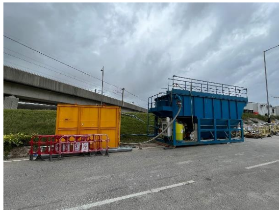
Setting up of sedimentation tanks for wastewater treatment facilities to increase the effectiveness of wastewater treatment
