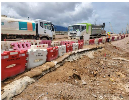
Sandbags were positioned underneath the water-filled barriers to prevent muddy water seepage out of the site boundaries
