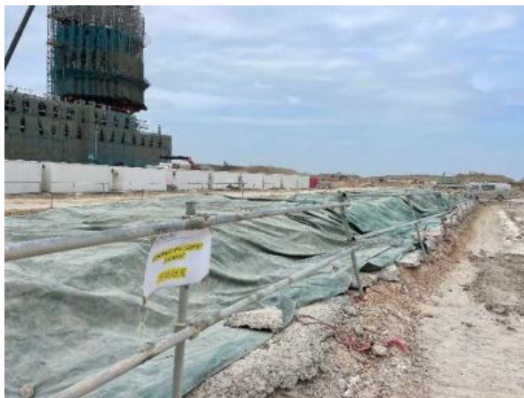
Excavated marine sediment is properly treated and reused as backfilling materials on site
