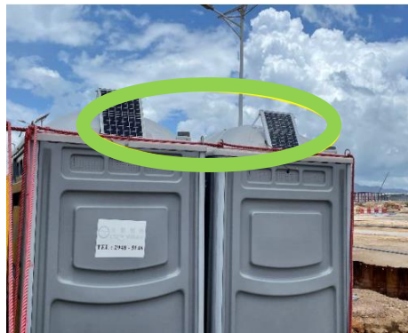
Use of renewable energy – solar lighting at mobile toilets
