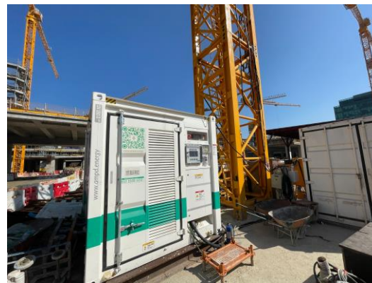
Use of renewable energy – use of battery energy storage for construction machines
