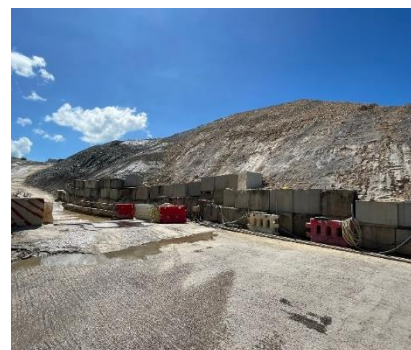
Concrete and excavated materials are properly segregated and stockpiled for reuse in land formation works
