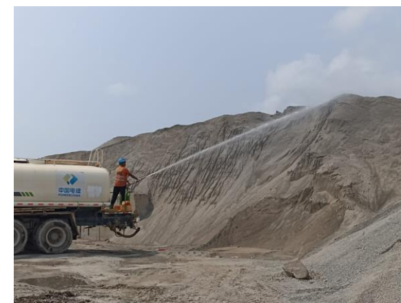
Regular water spraying for idled stockpile
