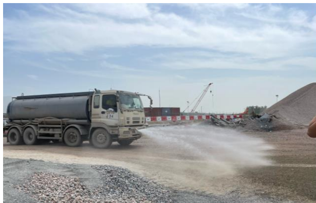
Regular water spraying at main haul road to minimise fugitive dust emission
