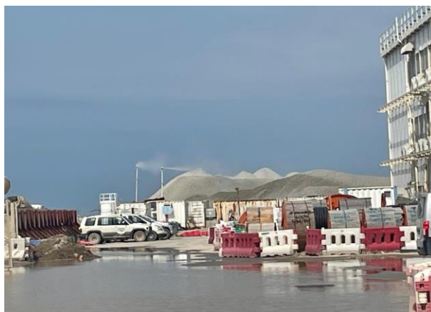
Automatic water sprinklers are installed at the stockpiling area
