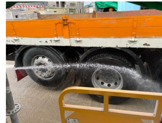
Setting up wheel washing facilities at site exits
