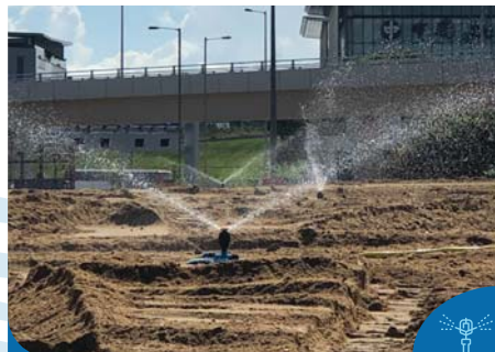
以360度自動花灑定期向填料灑水 Regularly using 360 degree automatic sprinkler to dampen fill materials
