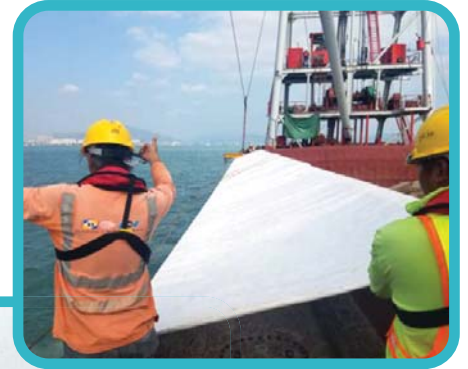
鋪設土工織物防護膜 Geotextile laying
