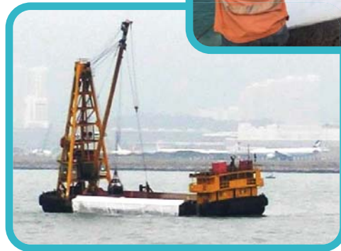
鋪設土工織物防護膜 Geotextile laying
