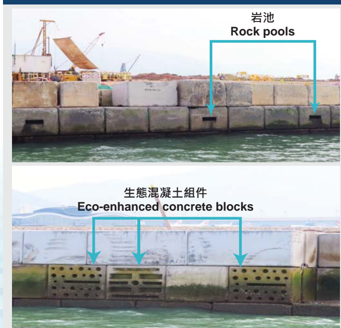
生態混凝土組件及岩池位於不同的潮汐水位，以助潮間帶和潮下帶生物在人工海堤上生長 Eco-enhanced concrete blocks and rock pools are located at different tidal levels to promote colonisation of intertidal and subtidal species on artificial seawalls
