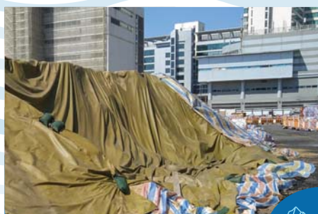
以不渗透的隔尘布覆盖储料区 Covering stockpiling areas with impervious sheets
