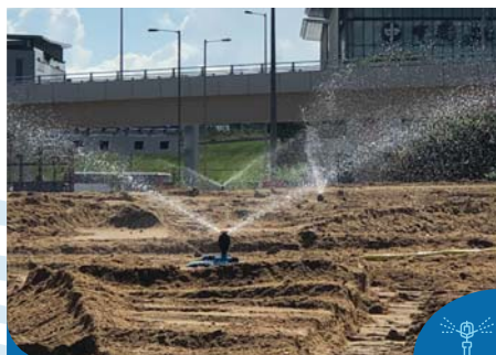
以360度自动花洒定期向填料洒水 Regularly using 360 degree automatic sprinkler to dampen fill materials
