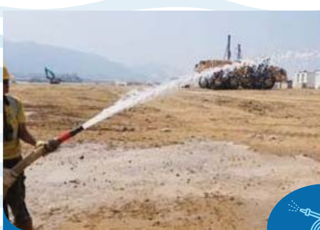
工人定时向工地洒水 Workers regularly hose works area
