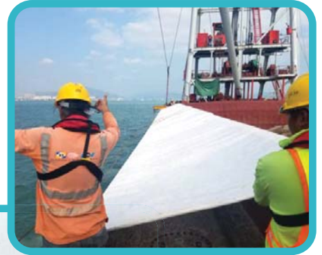
铺设土工织物防护膜 Geotextile laying
