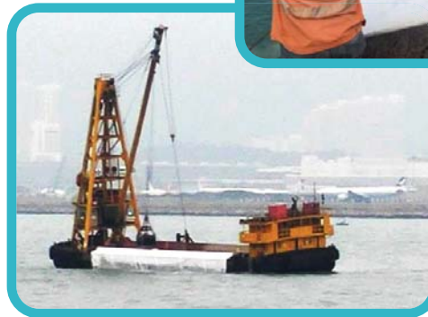
铺设土工织物防护膜 Geotextile laying
