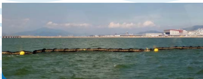
除局部设置的淤泥屏障外，在海上填料工程开始前於工地四周设置增强型淤泥屏障 In addition to localised silt curtains, enhanced silt curtain was deployed around works area before commencement of marine filling activities
