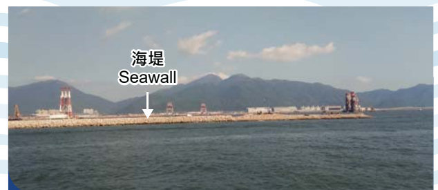
进行海上填料工程前先建造至少200米长的前缘海堤 An advance seawall of at least 200m was constructed prior to the commencement of marine filling activities
