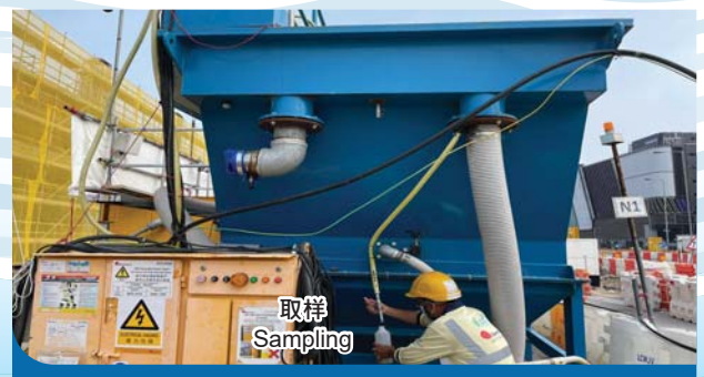
工地的污水在排放前须经污水处理设施处理，并定期由承建商取样监测，以确保符合《水污染管制条例》的要求 Wastewater discharged from construction site is processed at wastewater treatment facilities and monitored regularly by contractors to ensure compliance with the requirements of the Water Pollution Control Ordinance
