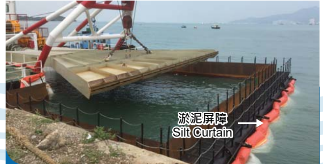
铺设砂垫层时设置笼式淤泥屏障 Deployment of localised cage-type silt curtains for sand blanket laying activities
