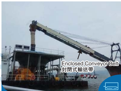
使用封閉式輸送帶運送填料 Using enclosed conveyor belt to transport fill materials
