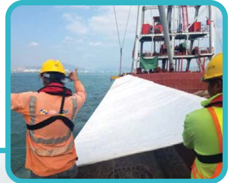
鋪設土工織物防護膜 Geotextile laying
