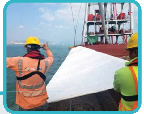
鋪設土工織物防護膜 Geotextile laying
