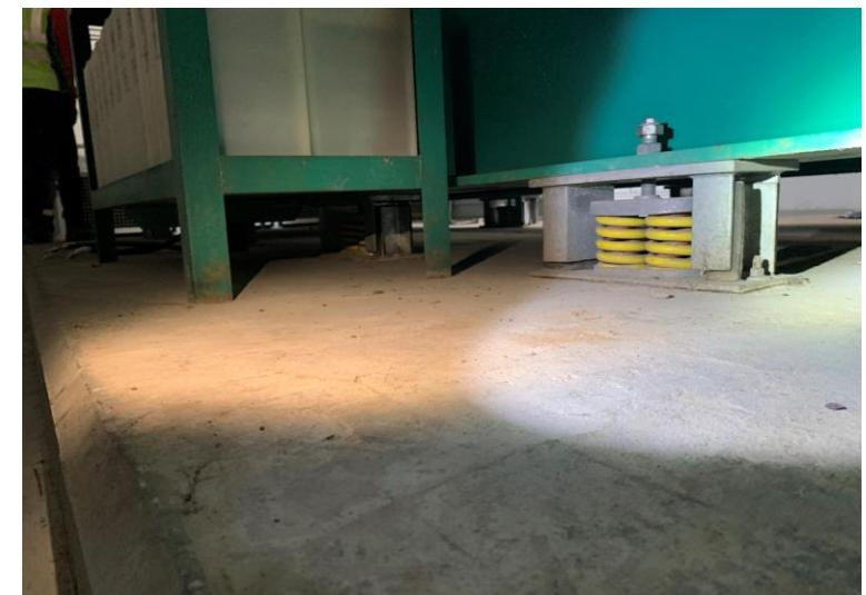
HS2 View 3 - concrete floor condition underneath emergency generator
