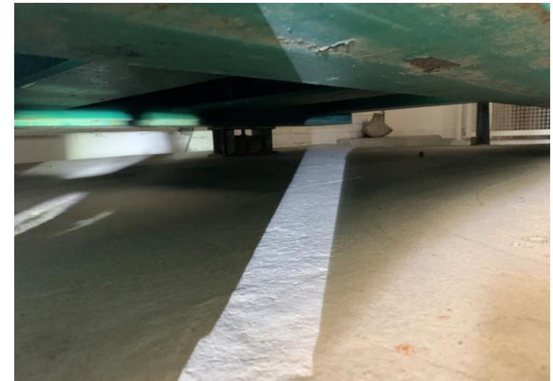
HS2 View 1 - concrete floor condition underneath emergency generator
