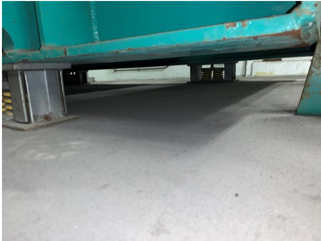
BH8 View 2 - concrete floor condition underneath emergency generator
