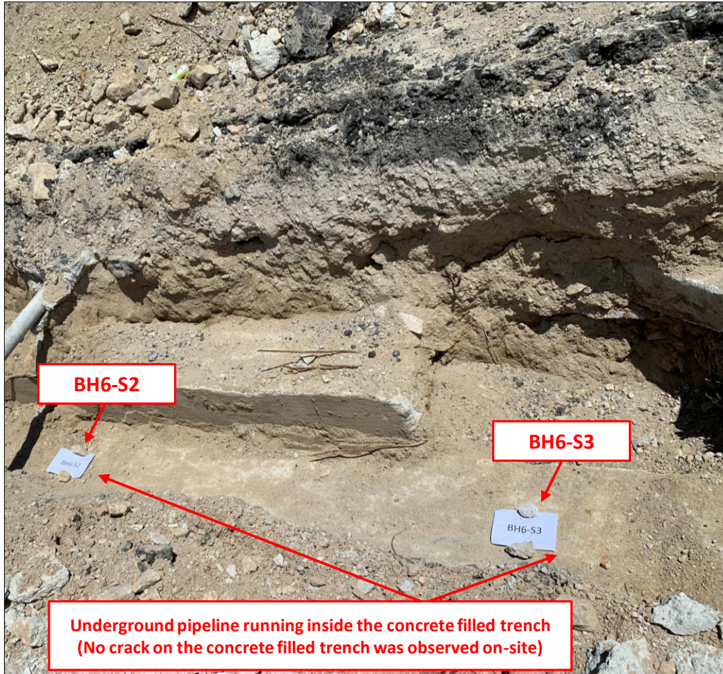
BH6-S2 and BH6-S3 View 1
