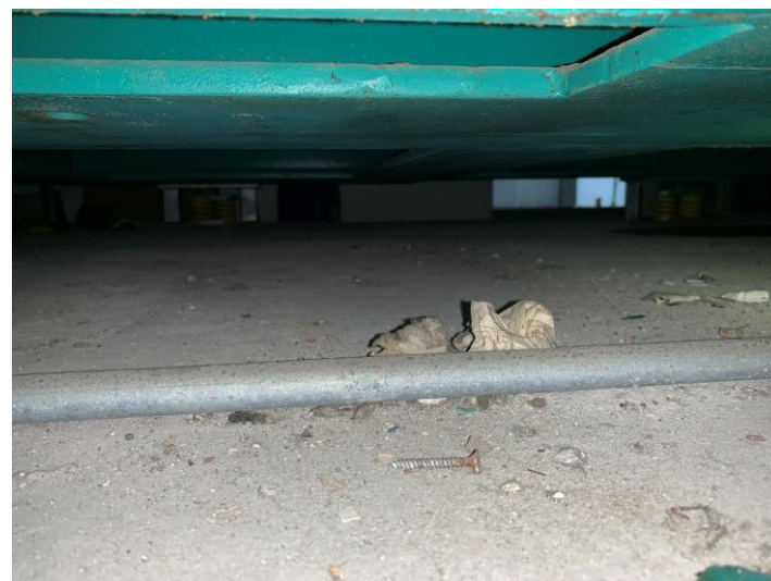
HS5 View 2 - concrete floor condition underneath emergency generator
