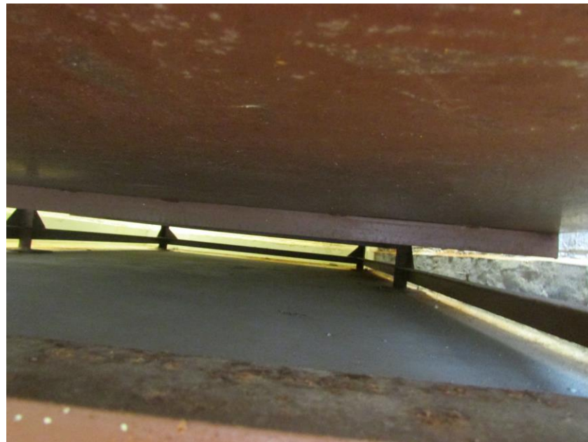
BH9 View 2 - concrete floor condition underneath 3000L Above-ground Fuel Tank
