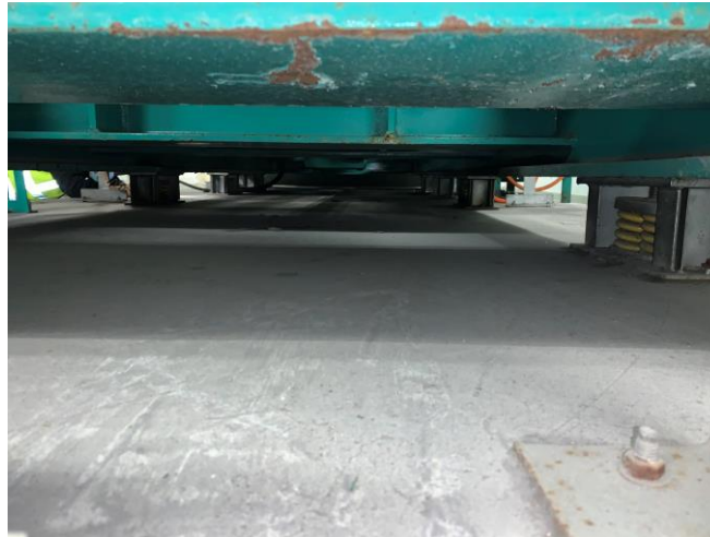
BH8 View 1 - concrete floor condition underneath emergency generator
