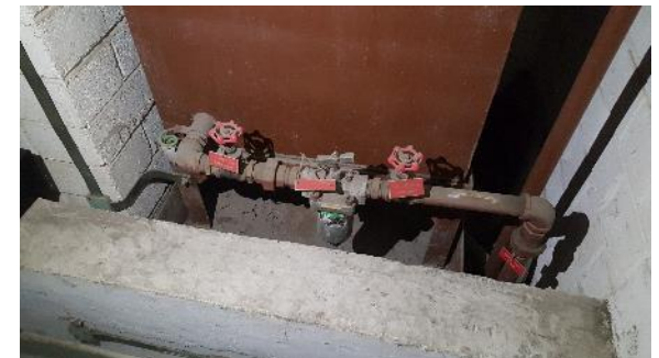
Metal drip tray and concrete curb surrounding fuel tank
