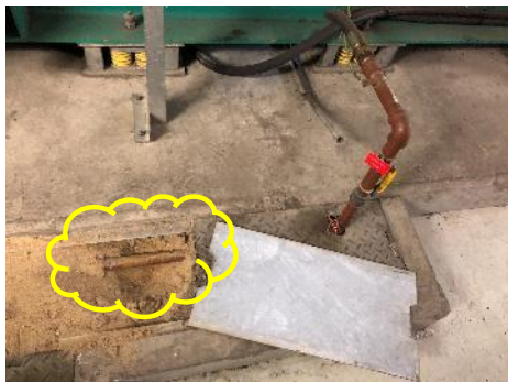
Exposed fuel pipes
