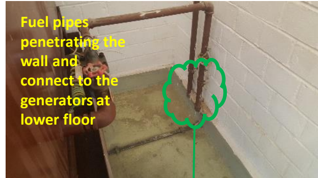
Fuel pipes penetrating the wall and connect to the 1500L fuel tank at upper floor
