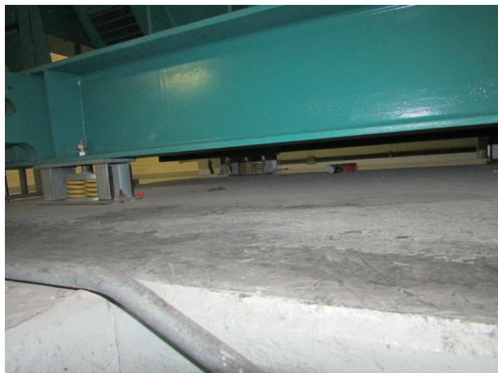
HS5 View 1 - concrete floor condition underneath emergency generator
