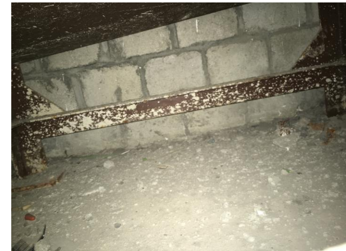
BH7 View 2 - concrete floor condition underneath 450 L Above-ground Fuel Tank
