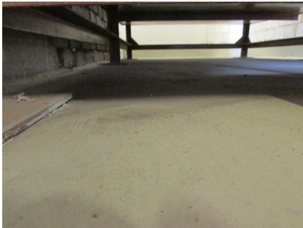
BH10 View 1 - concrete floor condition underneath 1,500L Above-ground Fuel Tank
