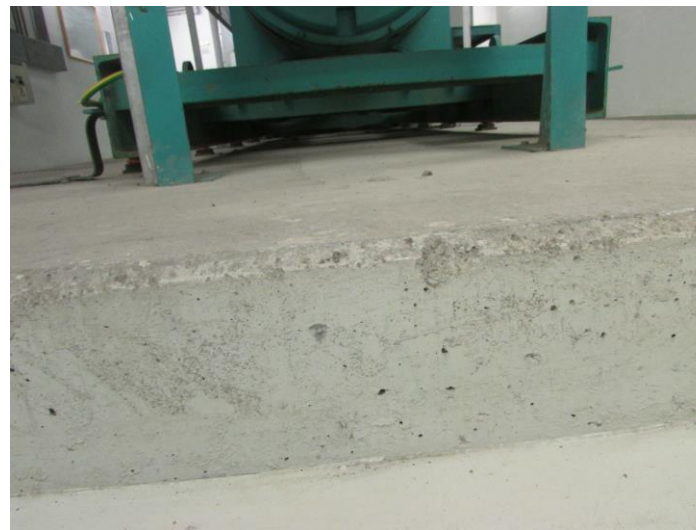
BH4 View 2 - concrete floor condition underneath Emergency Generator
