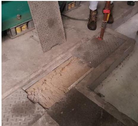
Sand filled trench containing fuel pipes (outside the fuel tank chamber)
