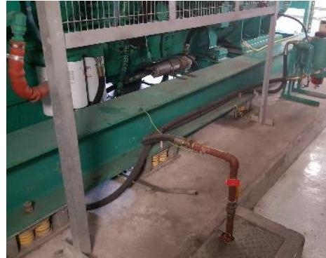
Fuel pipes to/from fuel tank and the generator
