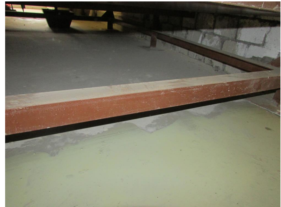
BH10 View 2 - concrete floor condition underneath 1,500L Above-ground Fuel Tank
