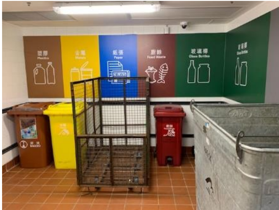
Figure 5.8 Recycling Facilities in Refuse room of the Passenger Terminal Building
