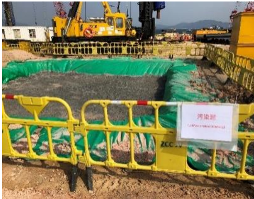
Use of impervious sheet to prevent potential seepage of contaminants from marine sediment to the surrounding
