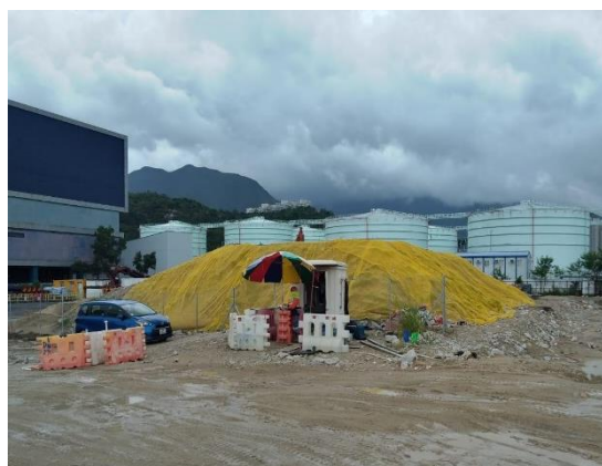
Covering the dusty stockpile with impervious sheet
