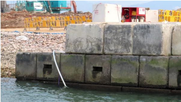
Since early 2020, 26 rock pool blocks installed (~100m)
