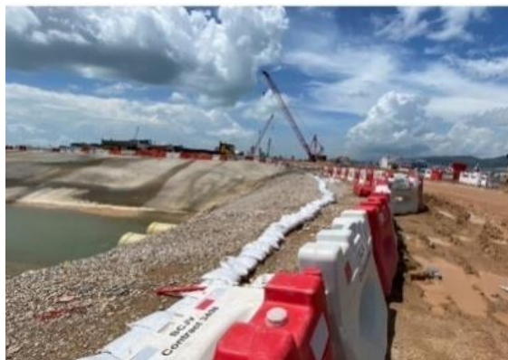
Provide sandbags and water-filled barrier to prevent direct discharge of muddy water into the marine environment.
