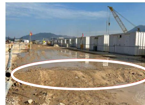
Provide earth bund as speed cushion to reduce fugitive dust generation.
