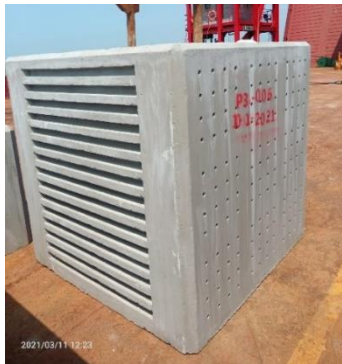
46 three-surfaced eco-blocks were installed at the northeast of 3RS Project area (~ 2,200m)
