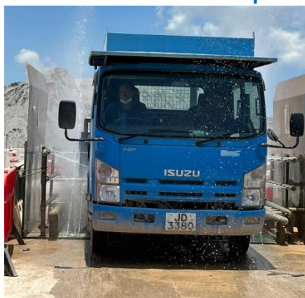
Install wheel washing facilities with high pressure water jet at site exit to avoid carrying of dust and soil to public road by site vehicles
