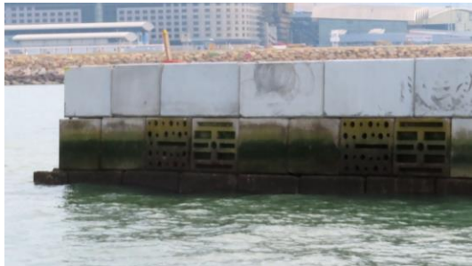
Since early 2020, 116 eco-enhanced concrete blocks installed (with a length of around 330m)
