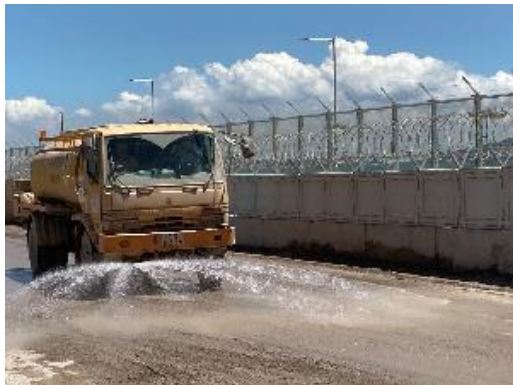
Provide regular water spraying at the main haul road to reduce fugitive dust generation.
