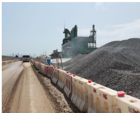
Provide water spraying on dusty stockpile by 360° automatic water sprinklers
