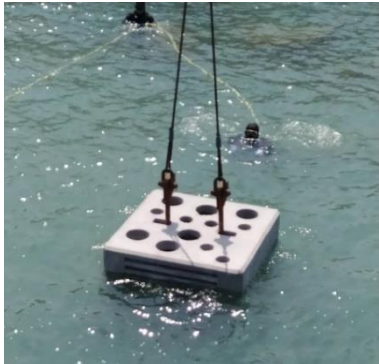
46 three-surfaced eco-blocks were installed at the northeast of 3RS Project area (~ 2,200m)
