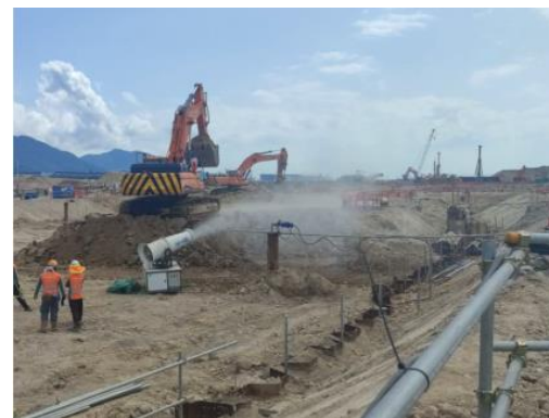
Provide regular water spraying on dusty stockpile by mist cannon
