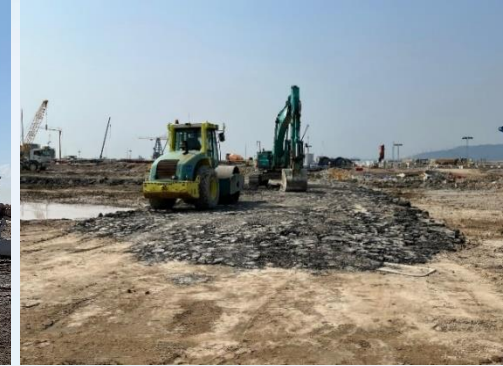
Reuse of asphalt for paving main haul roads
