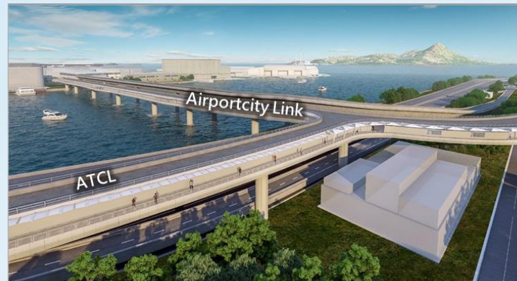
Integrates with Airportcity Link to form an autonomous transportation system
