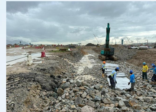
Reuse of armour rocks for land formation works
