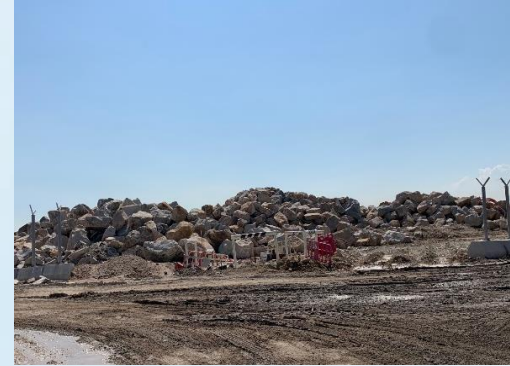
Excavated materials are segregated and stockpiled for reuse
