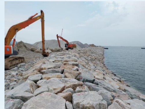
Reuse of armour rocks for seawall construction
