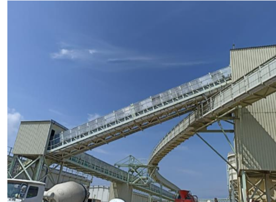
Conveyor belts were fully enclosed to prevent fugitive dust emission
