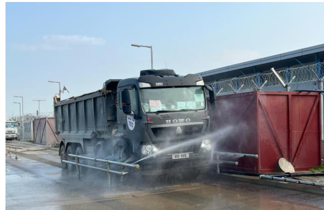
Install wheel washing facilities with high pressure water jet at site exit to avoid carrying of dust and soil to public road by site vehicles
