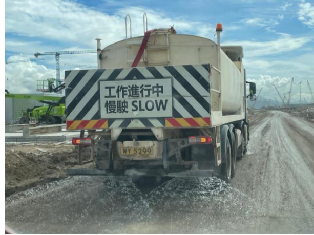
Regular water spraying at haul roads to reduce fugitive dust emission
