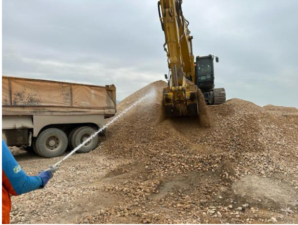
Regular water spraying at stockpiles to reduce fugitive dust emission
