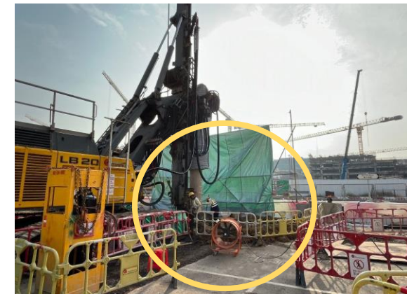
Curtains were erected next to works areas to reduce dust nuisance
