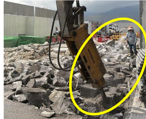
Water spraying during breaking activities to minimise dust emissions
