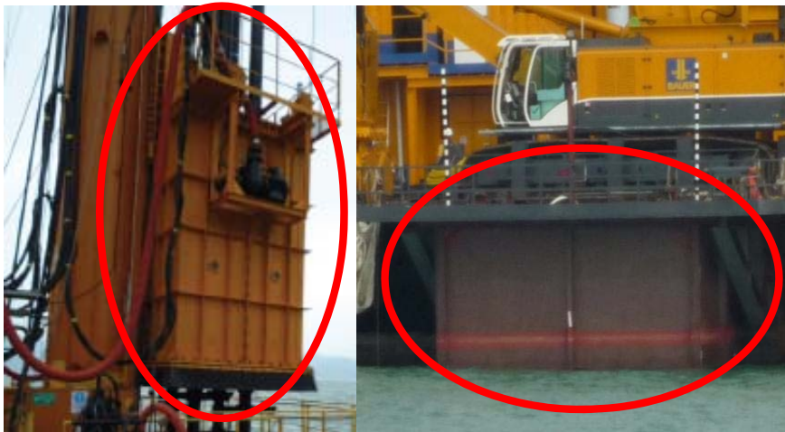
1. Silt Curtain Surrounding DCM Mixing Shaft
