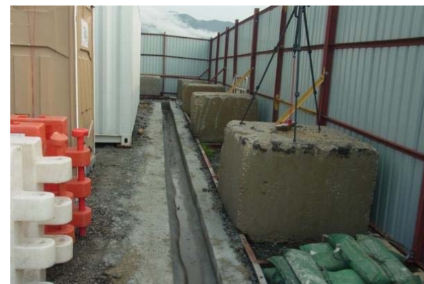
Installation of u-channel for site drainage
