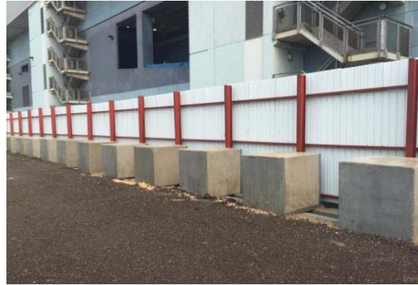
Erection of hoarding along site boundary
