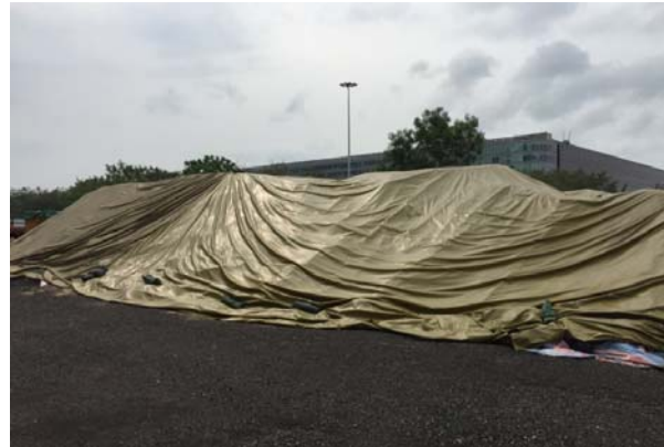
Cover excavated materials by tarpaulin to prevent dust generation
