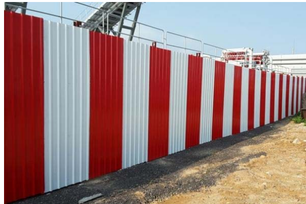
Erection of hoarding along site boundary
