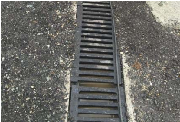
Installation of u-channel for site drainage
