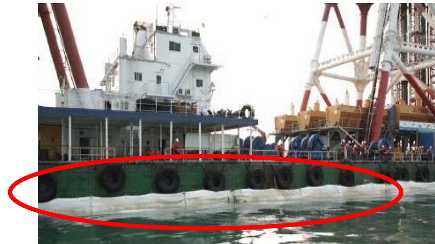
2. Silt Curtain Surrounding DCM Barge / Works Area in case of emergency
