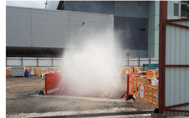
Provide wheel washing facility to remove any dusty materials from vehicle body and wheels
