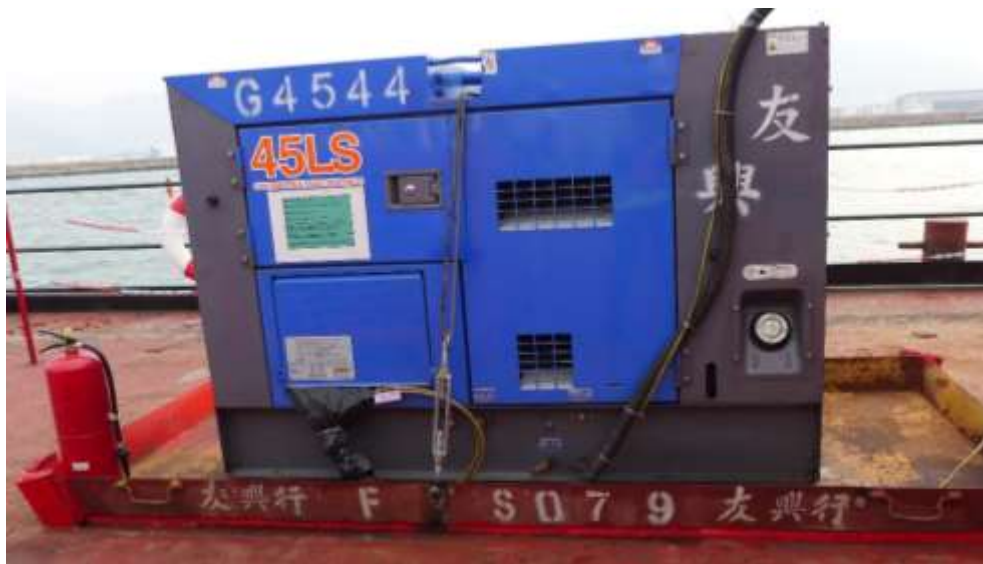
Full enclosure of generator set/ compressor
