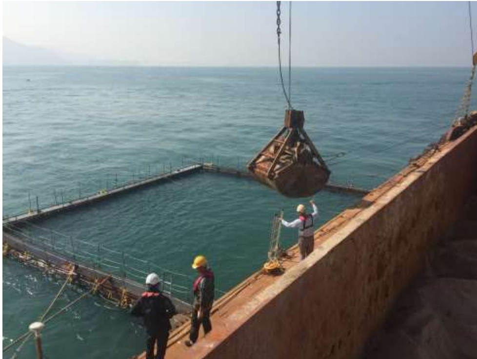
Deployment of silt curtain for sand blanket laying
