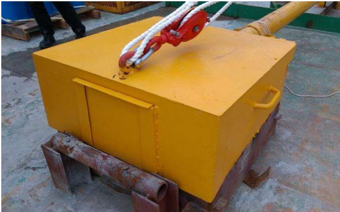
Enclosure at cement connecting pipes to minimise dust dispersion
