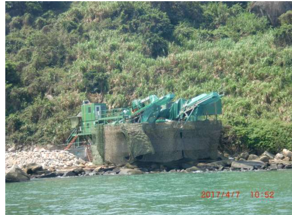
Checking of containment pit on Sheung Sha Chau for prevention of any effluent discharge to surrounding waters
