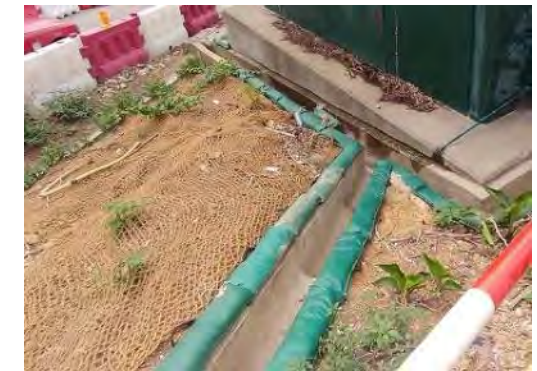
Sandbags serve to protect channels from surface runoff
