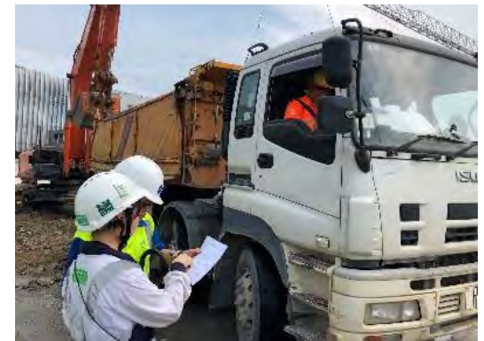
Checking of records presented by truck driver on delivery of construction and demolition (C&D) waste
