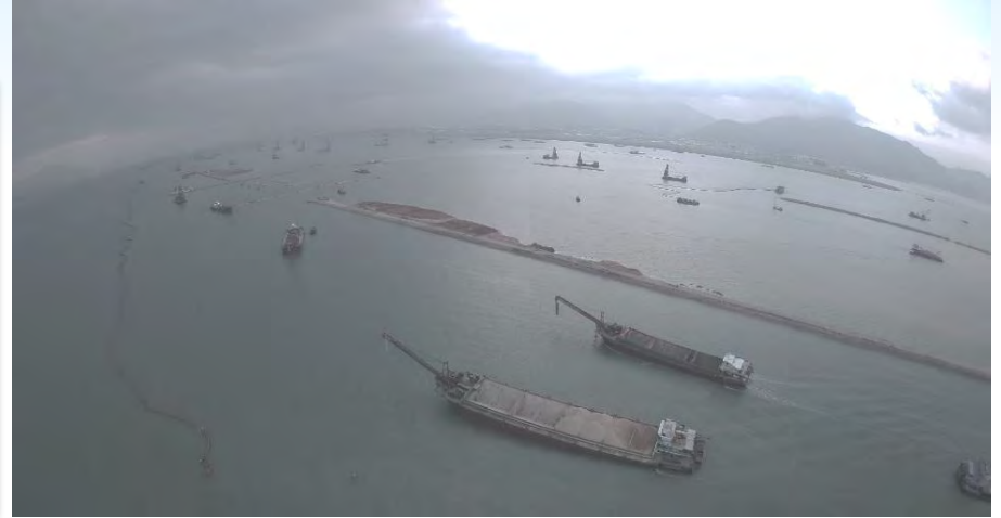
Seawall construction and filling activities
