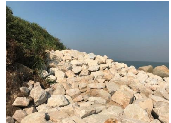
Rockfill reused for shoreline reinstatement on Sheung Sha Chau
