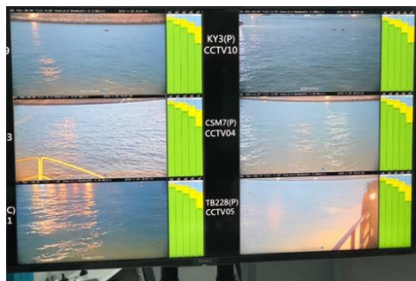
CCTV system for DEZ monitoring
